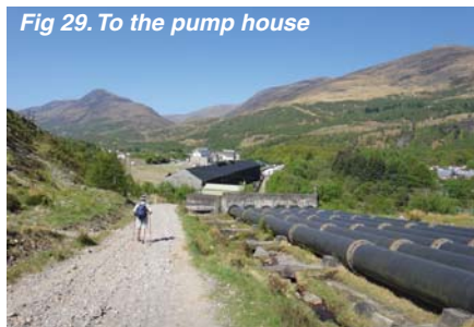
Fig 29. To the pump house
